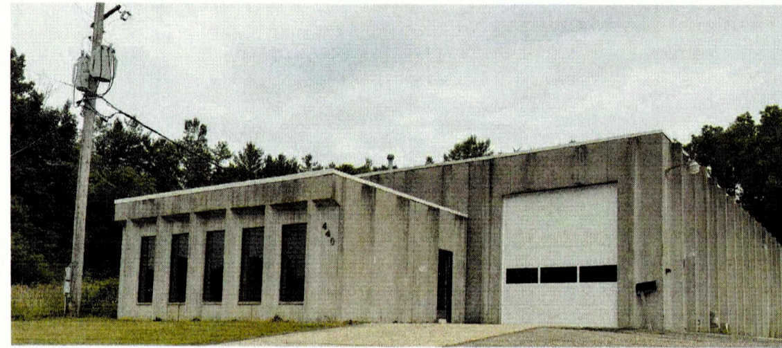
FRONT ELEVATION FROM SOUTH STREET
