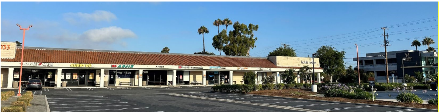
3. Remaining portion of existing multi-tenant building - facing Bristol Street
