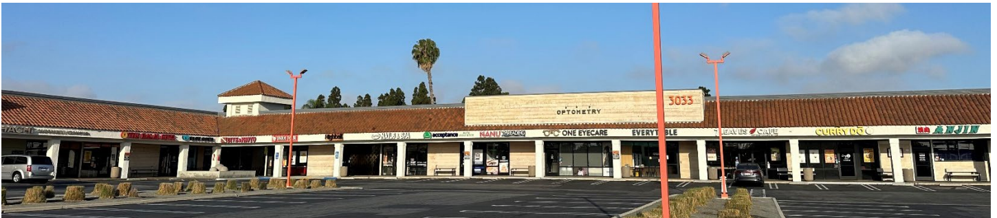
2. Portion of existing multi-tenant building - facing Bristol Street
